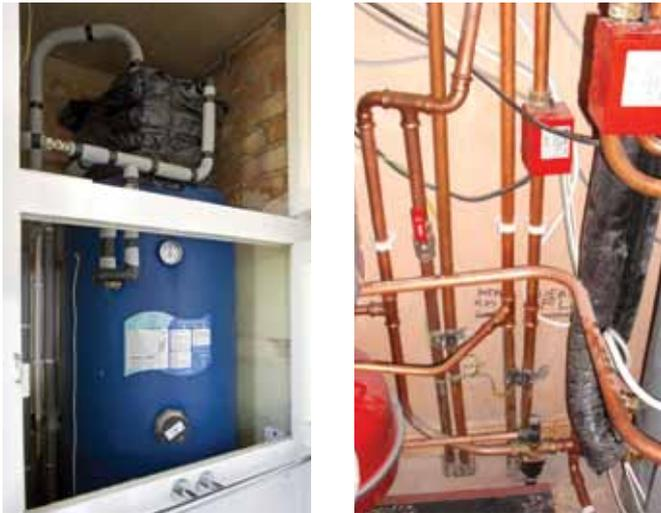
**Figure 8. Two solar water heating systems showing good (left) and poor (right) levels of insulation**
